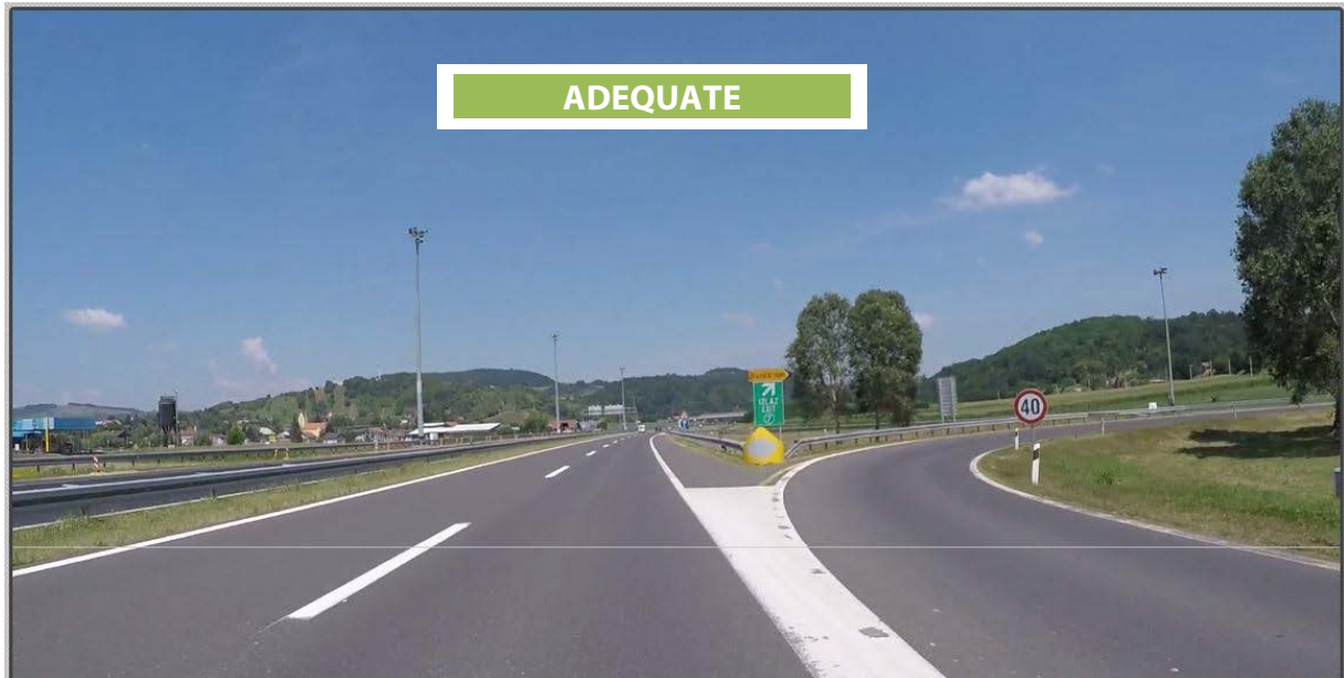
Segment 431667 at A4_Breznicki_Hum_Novi_Marof_A Road (id 403)
